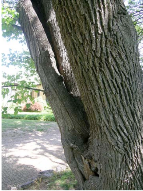
Figure 89. Elm with deep-seated hollows on branch and trunk
